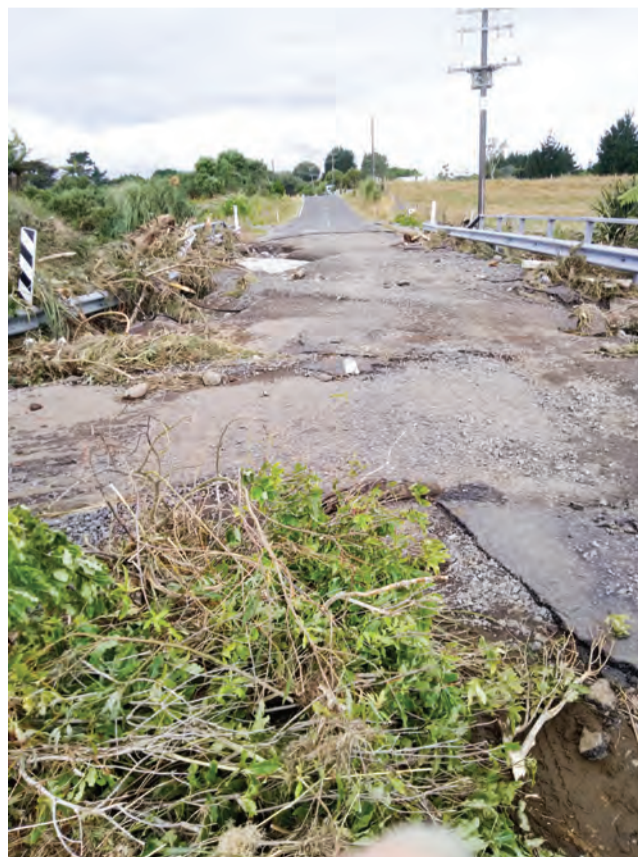
The Mid-Parihaka Road bridge was rendered impassable.
