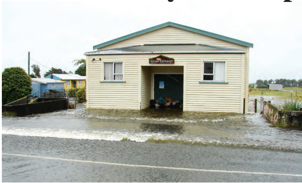
This building was sandbagged in an attempt to stop floodwaters from coming inside.
